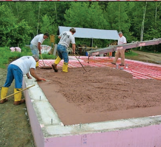
Step 7: The medium-brown integral color used to tint the concrete will help absorb solar radiation efficiently.
