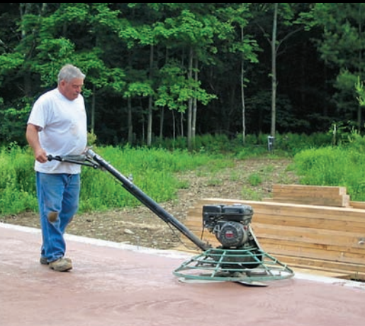
Step 9: Power-troweling the slab provides a smooth finish.
