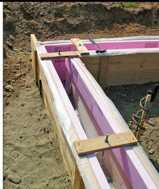
Step 1: Frost-protected shallow (FPS) foundation with exterior and slab-edge insulation pre-installed.
