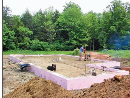
Step 3: Leveling and compacting the subslab fill.
