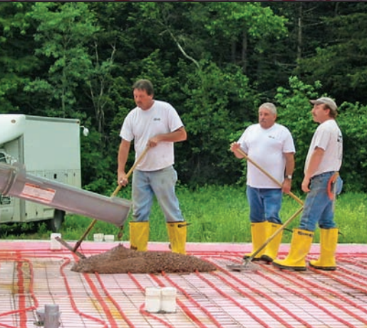
Step 6: Pouring and distributing the concrete.
