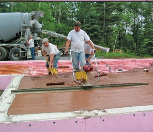
Step 8: Smoothing the slab's surface to its final texture.
