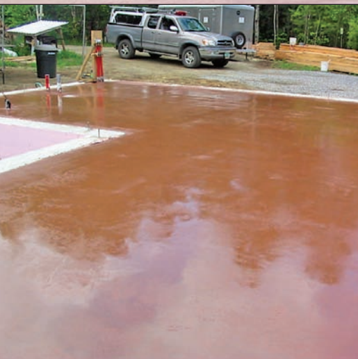
Step 10: Applying a curing sealer over the finished concrete will help protect the surface from stains.
