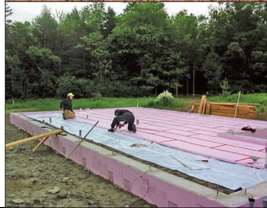
Step 4: With the vapor barrier installed, a layer of rigid foam insulation over it provides a thermal break from the earth.
