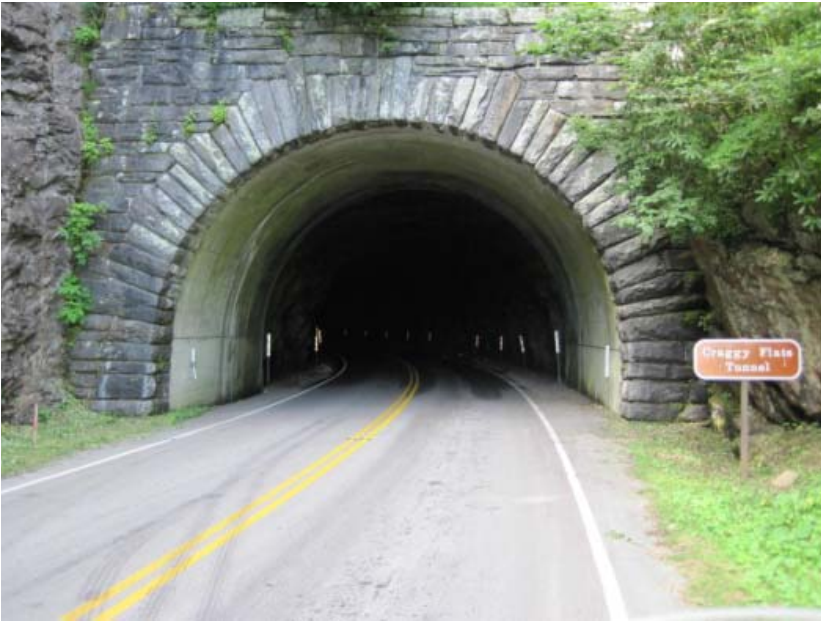
Blue Ridge Parkway Tunnel
