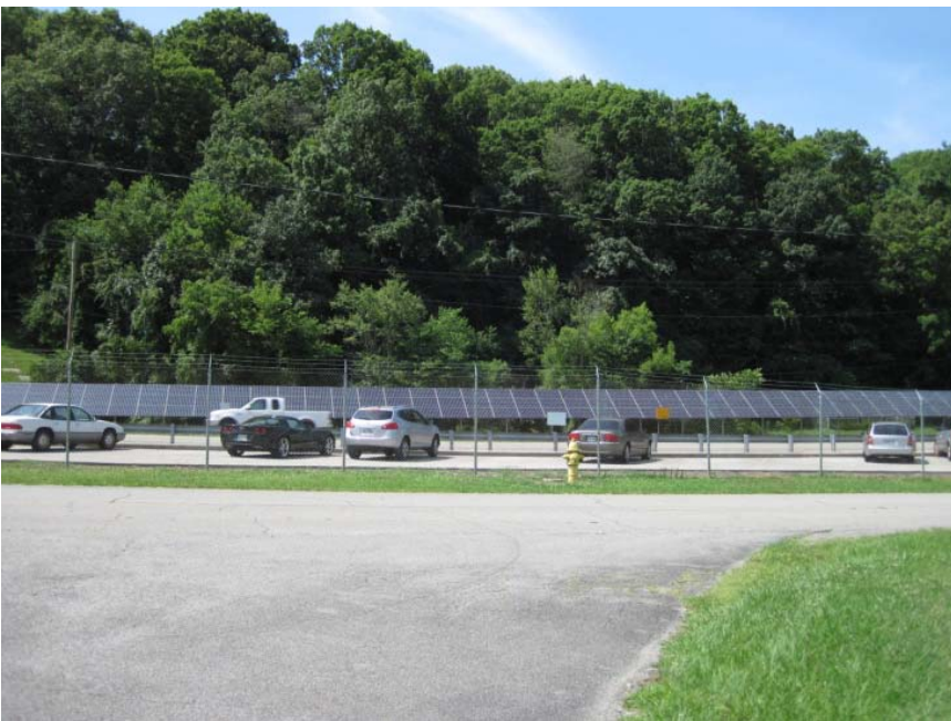
Solar array powers building at
